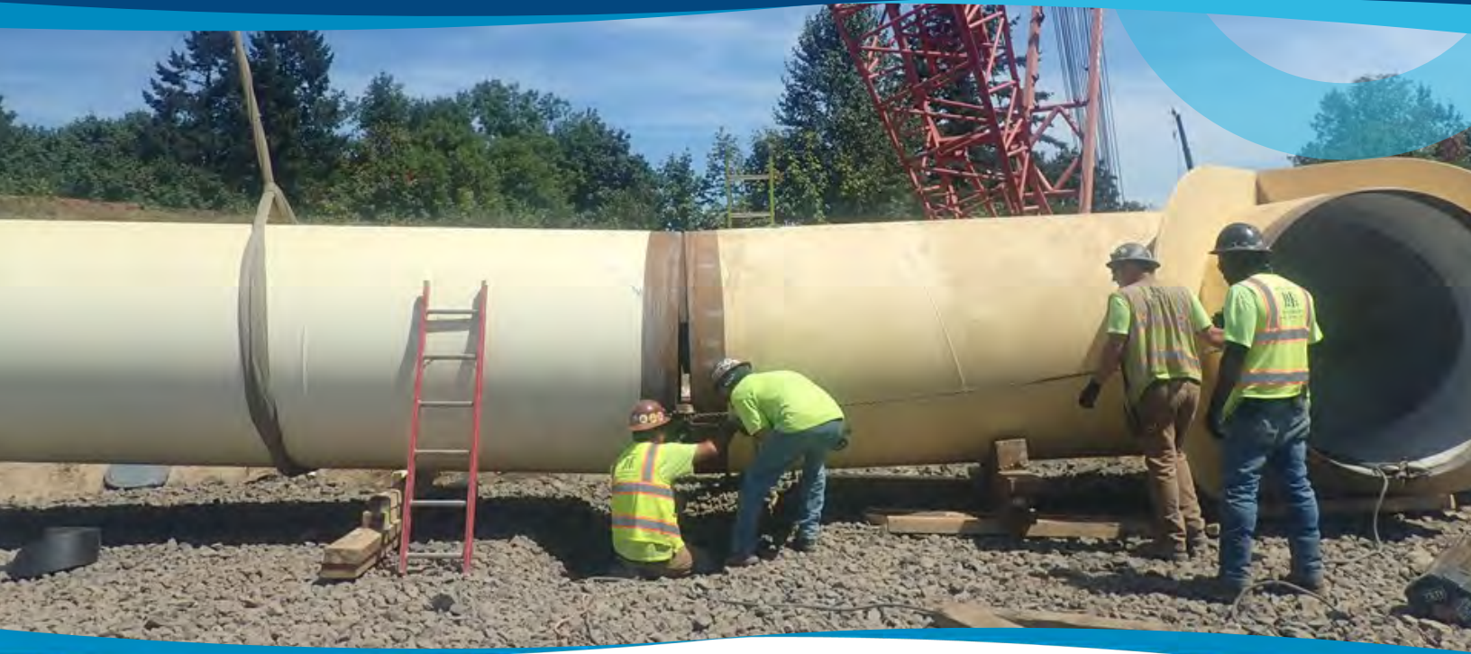
Willamette Water Supply System large diameter pipe installation
