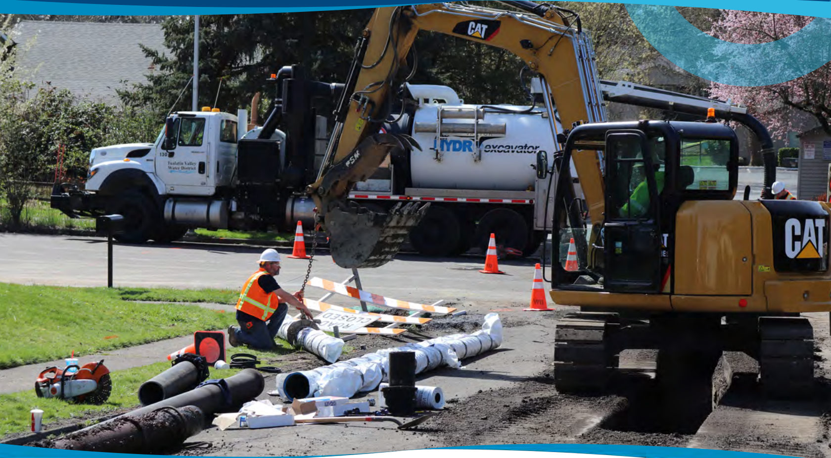
Water main replacement
