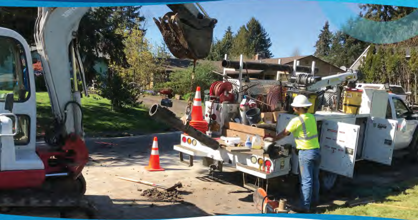
Operators replace a broken water main
