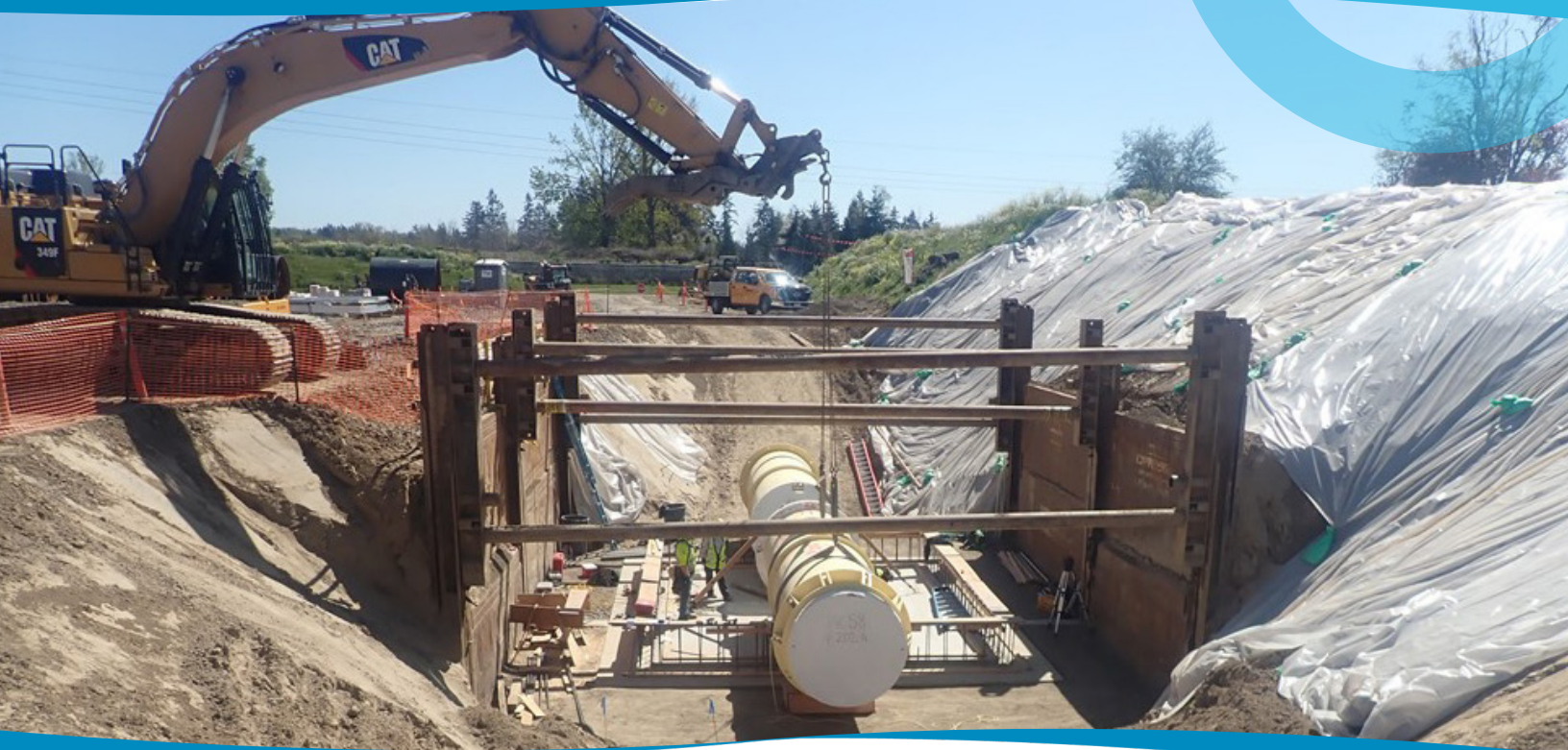
Pipe installation for the Willamette Water Supply System
