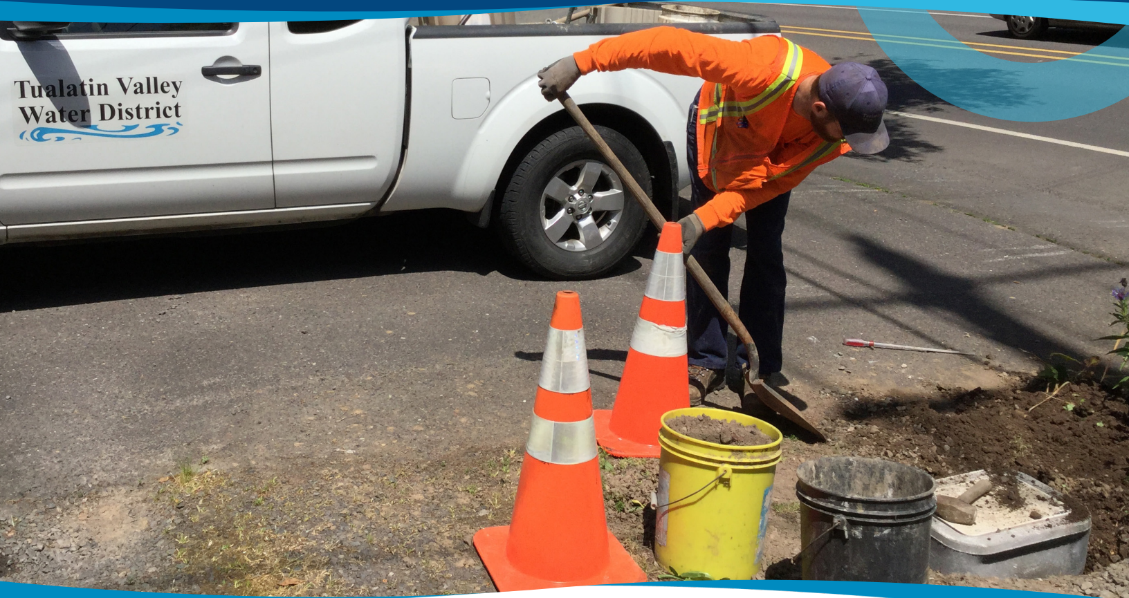
A District employee finishes a water meter repair
