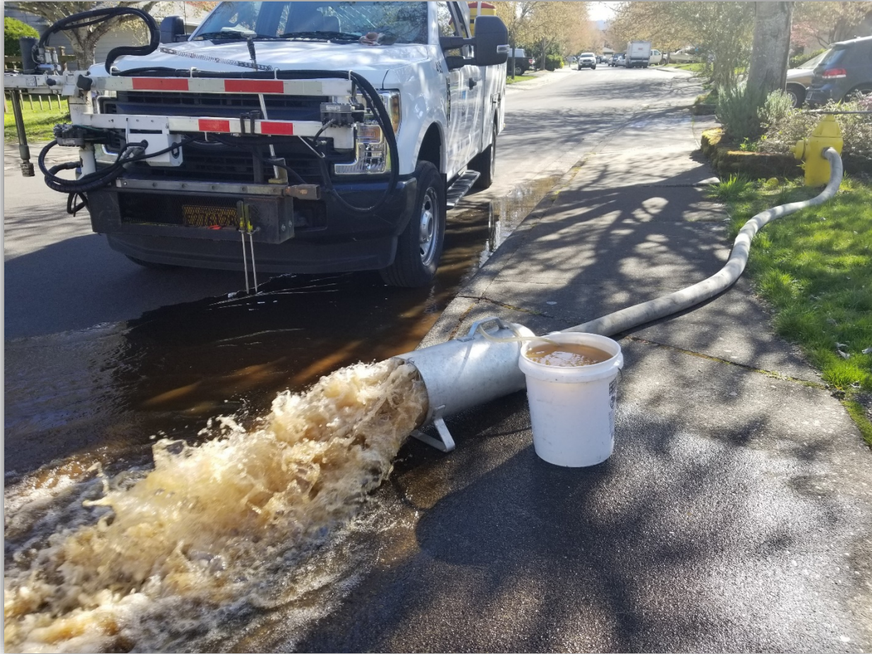
Flushing to remove sediments and manage water age
