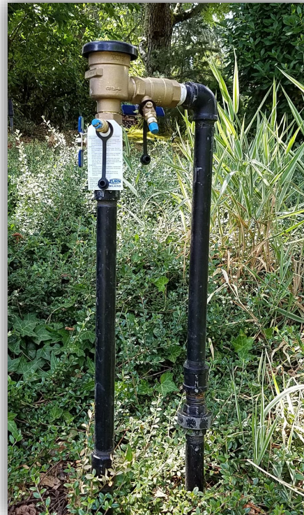
Pressure Vacuum Breaker Assembly (PVB)
