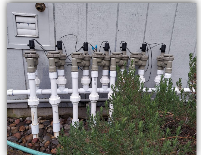
Atmospheric Vacuum Breaker (AVB)
