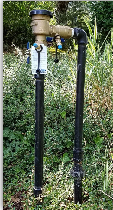
Pressure Vacuum Breaker Assembly (PVB)
