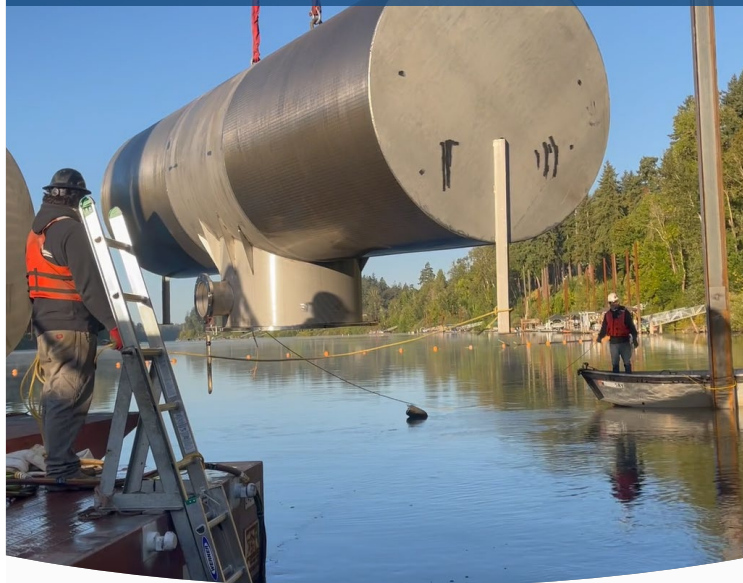
Willamette Intake Facilities fish screen replacements (Sept 2021)
