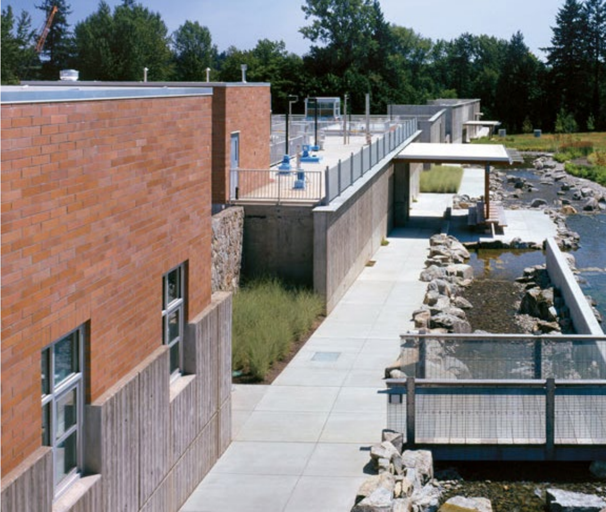
Willamette River Water Treatment Plant
