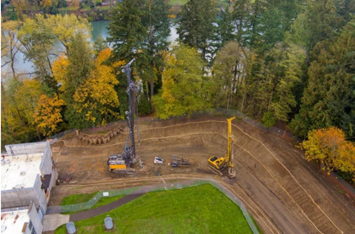
Deep Soil Mixing
