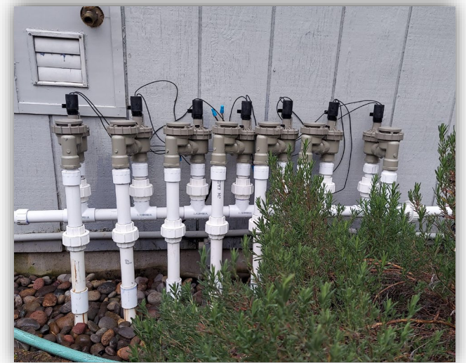
Atmospheric Vacuum Breaker (AVB)
