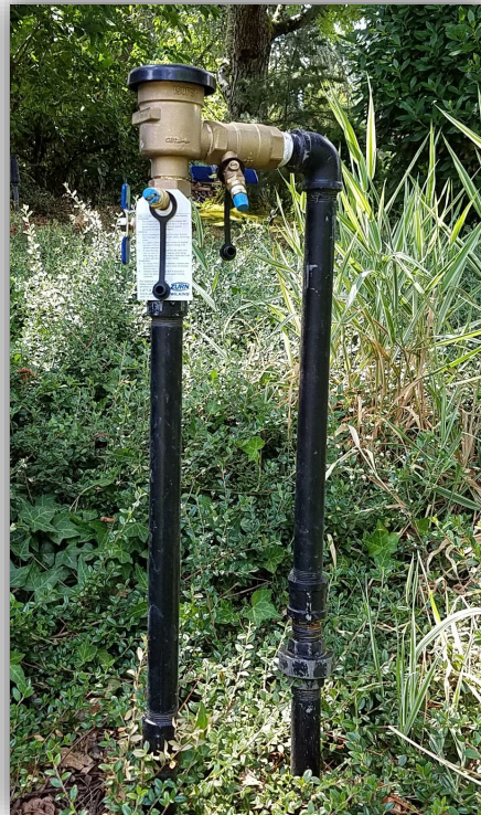
Pressure Vacuum Breaker Assembly (PVB)
