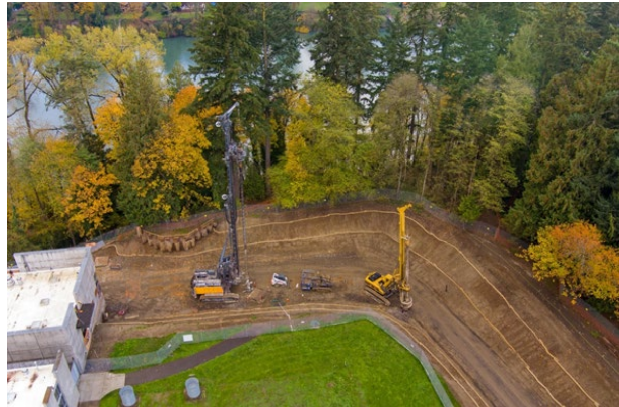
Deep Soil Mixing
