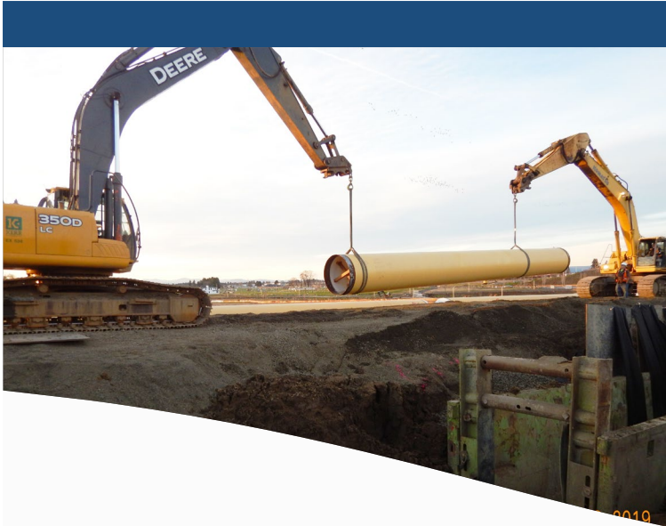
Construction of the additional water supply
