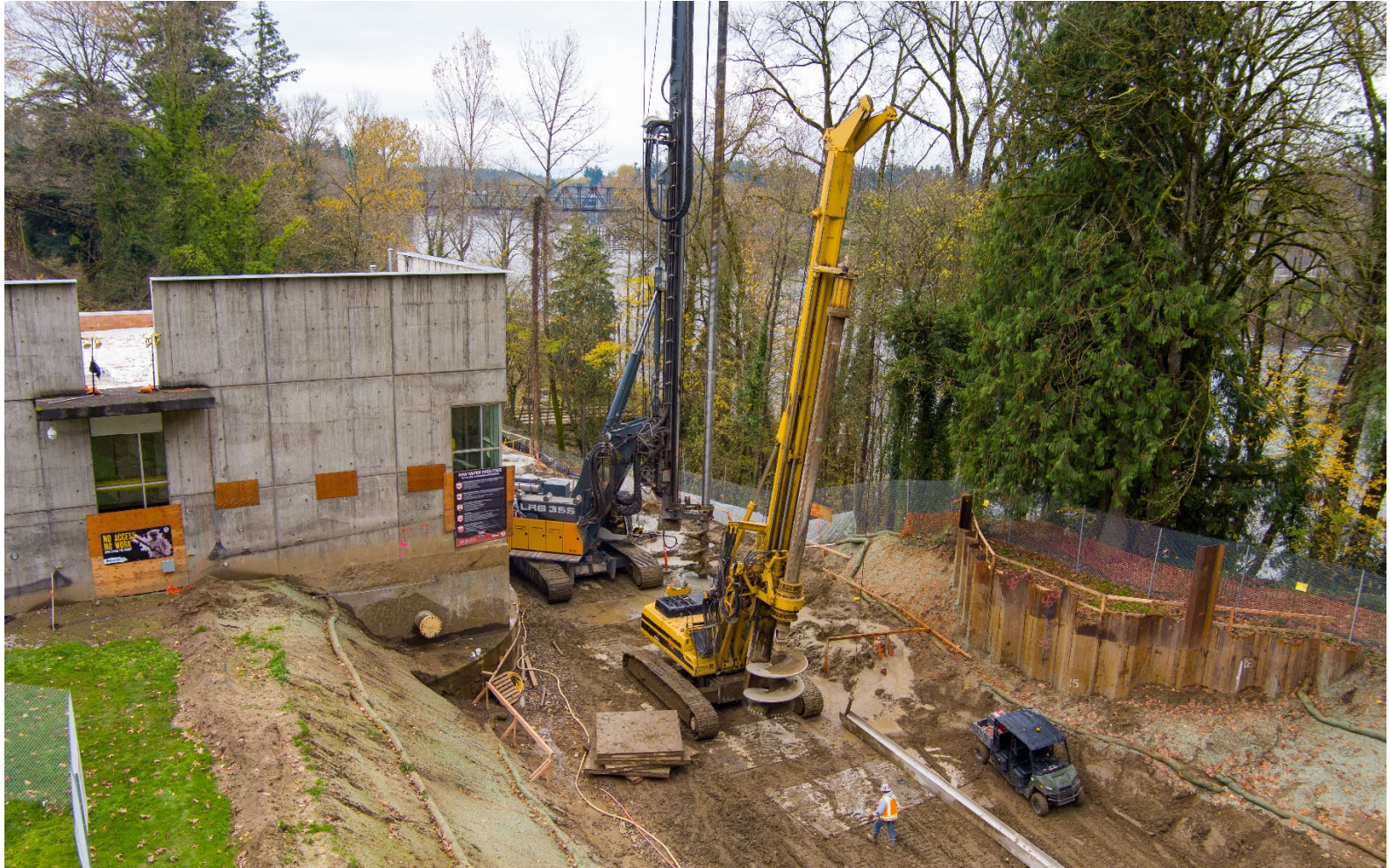
Seismic improvements at the river intake
