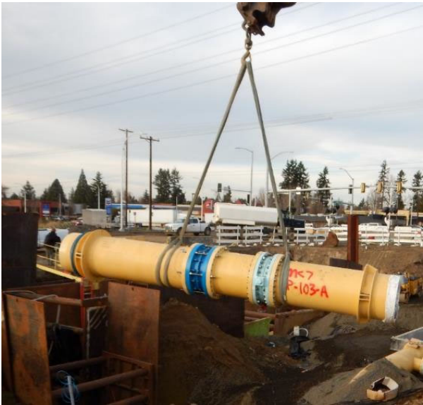
South Hillsboro Area Pipeline Project Coordinated with Newland
