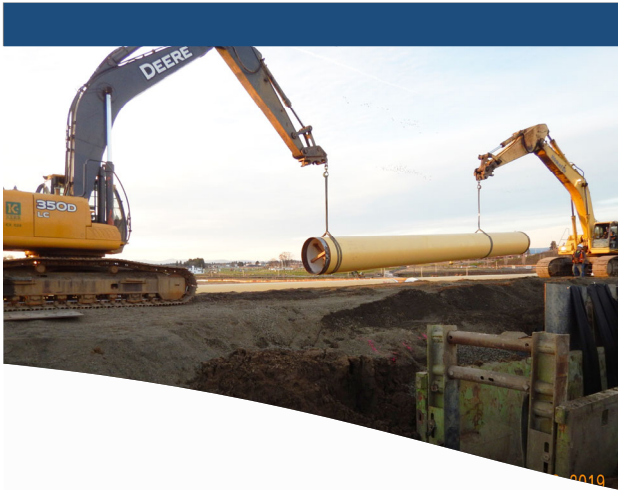
Construction of the additional water supply
