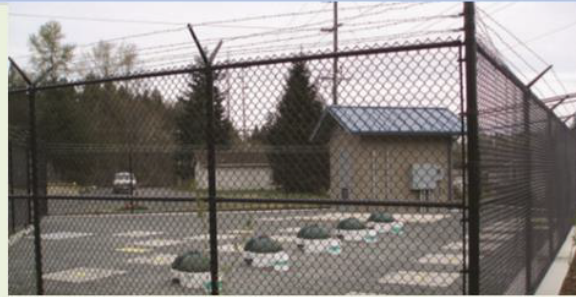
Image: Example pump station
