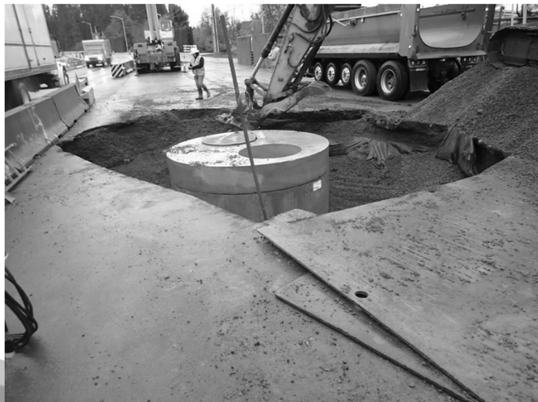
Installing access vault near Chicken Creek and Roy Rogers Rd.
