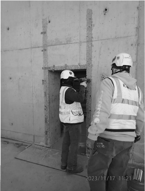
Slide gate installation at EQ Basin
