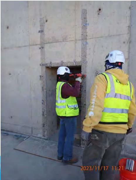
Slide gate installation at EQ Basin
