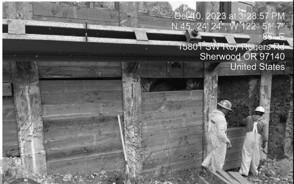
Installation of retaining wall at Tributary #4
