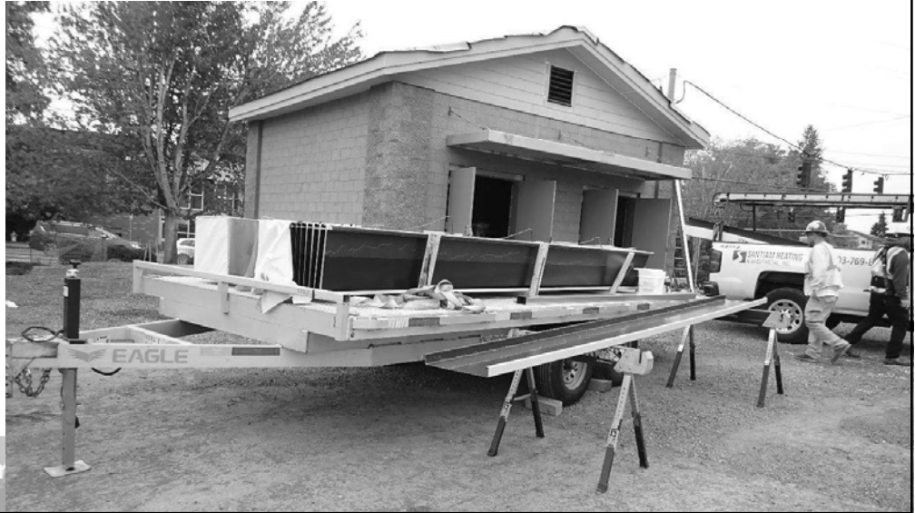
PFC Building roof installation
