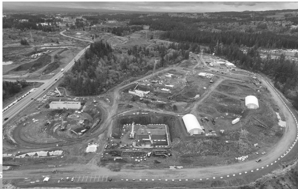
WTP site looking south
