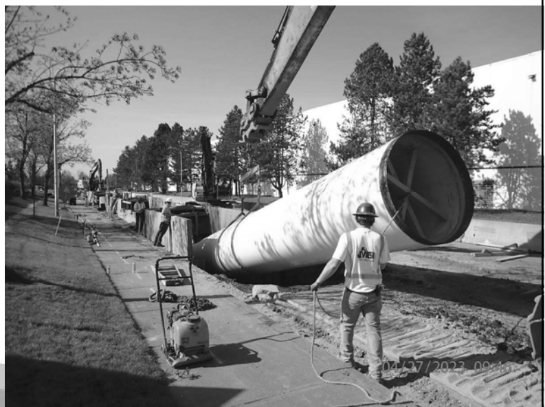
66-inch pipe installation on 95 th Avenue
