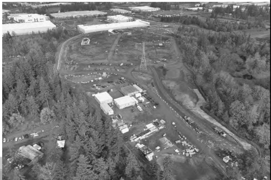
WTP site looking northwest
