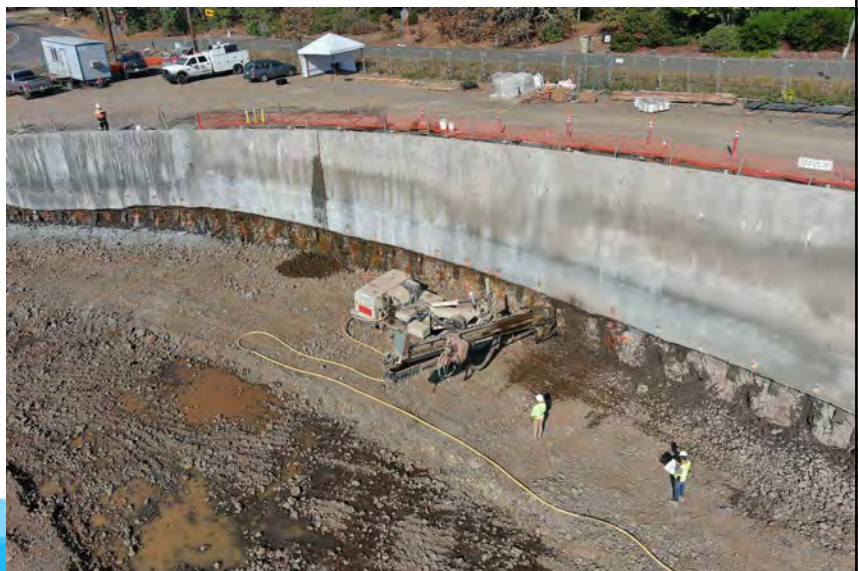
Retention wall RES_1.0 site
