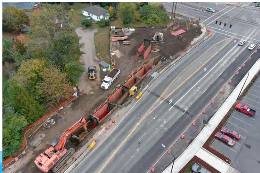
66" pipe installation along north side of Roy Rogers
