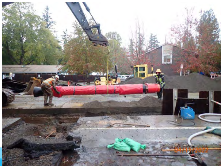
Installation of COB ductile iron pipe on Denney Rd.
