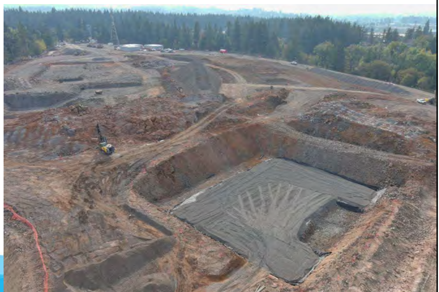
EQ basin area subgrade preparation
