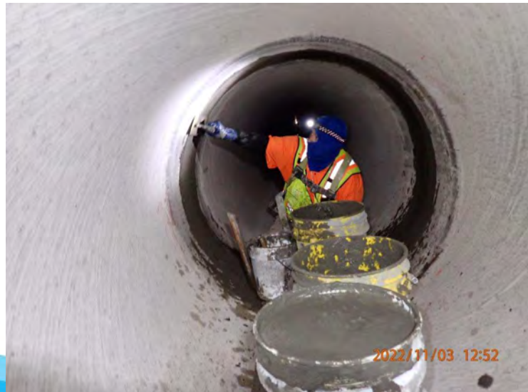
48" WWSP waterline joint grouting
