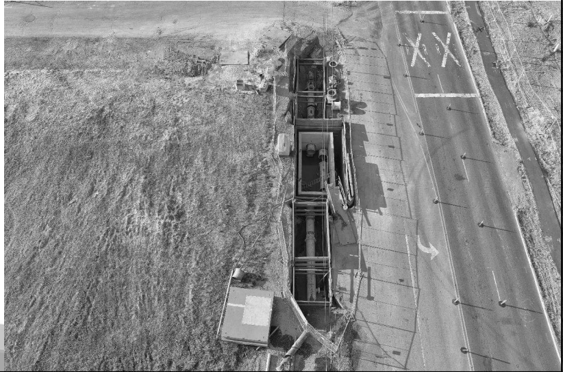
Flowmeter vault construction
