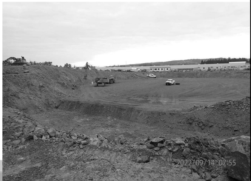
Looking north: Clearwell and Pump Station subgrade prep
