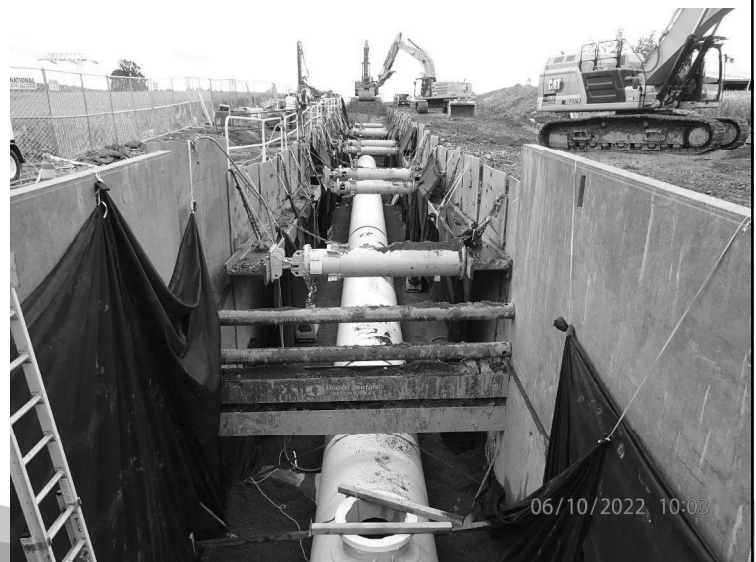
66-inch waterline installation
