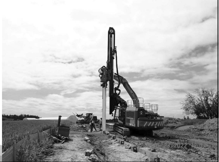
Shoring installation for 66-inch waterline installation
