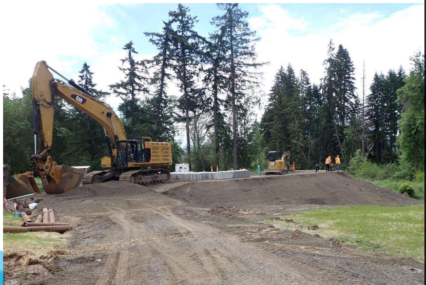
Graded pad at north side of Butternut Creek
