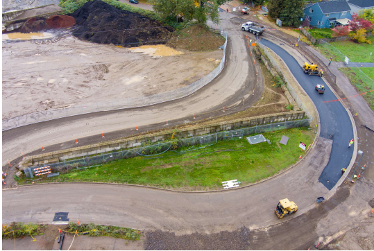
Pinch point pavement replacement
