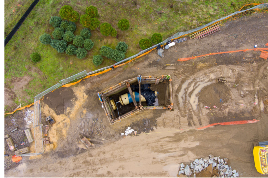
Connection to adjacent PLM_1.1 pipeline
