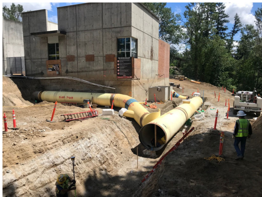
New WWSS header and cut and cap of existing WRWTP header
