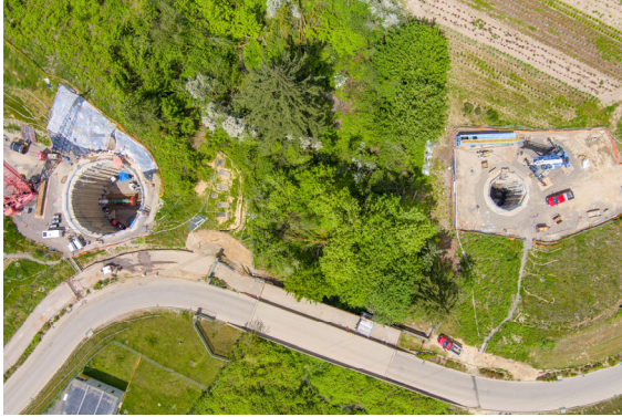
Trenchless crossing launching and receiving shafts
