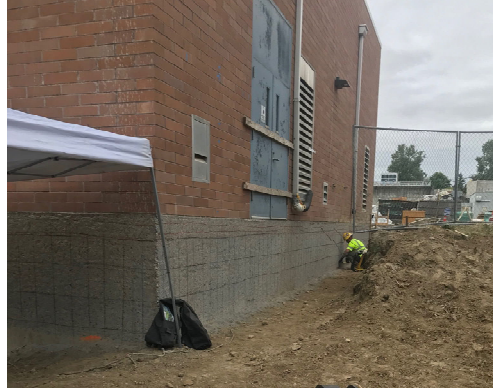
Seismic improvements at RWPS
