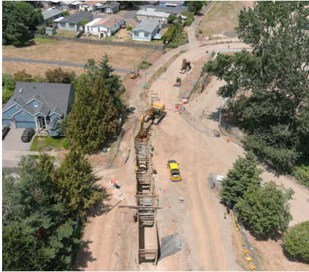
Shoring for pinch point
