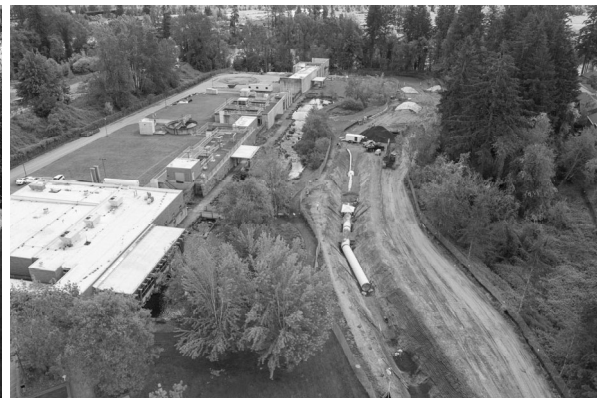
66" pipe in Park
