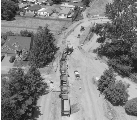
Shoring for pinch point
