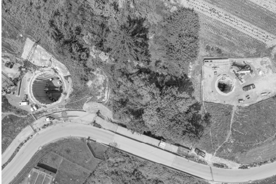
Trenchless crossing launching and receiving shafts
