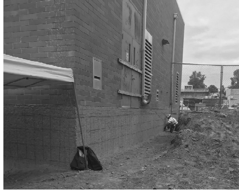
Seismic improvements at RWPS
