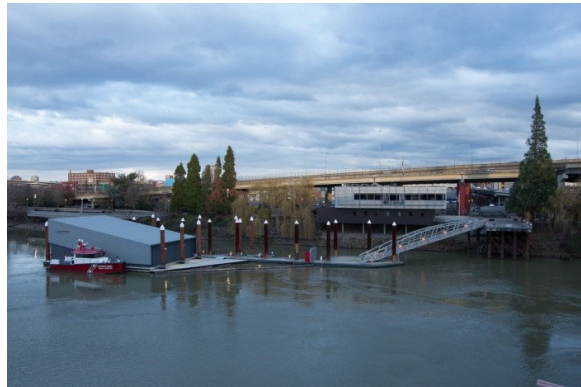
Firehouse No.21 on Willamette River
