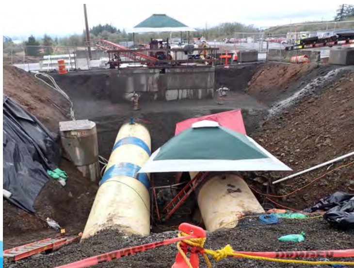
66-inch inlet and outlet waterline tie-in from reservoir site to PLM_5.3
