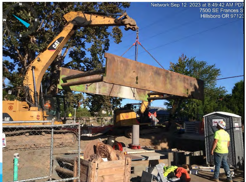
Frances Street turnout vault and piping construction
