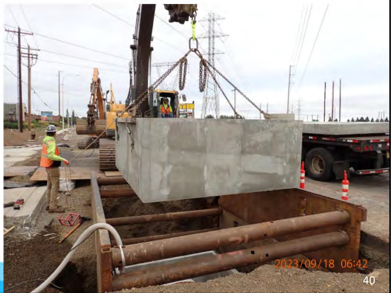
Setting precast concrete access vault.
