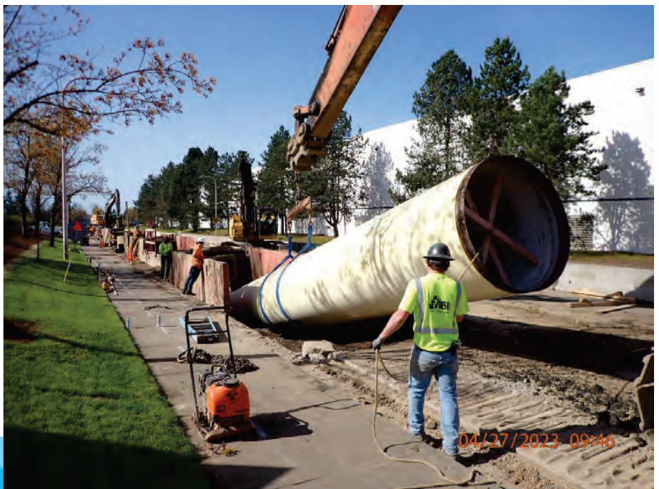
66-inch pipe installation on 95 th Avenue
