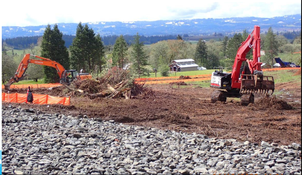
Grubbing on Staging Area #1
