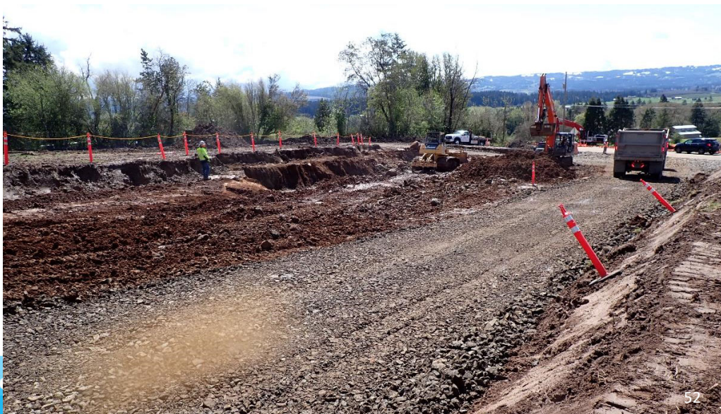
Initial earthwork at RES site
