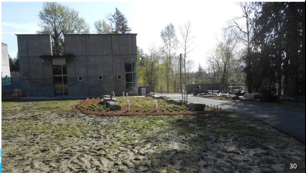
Raw Water Pump Station, Main Overlook, landscaping
