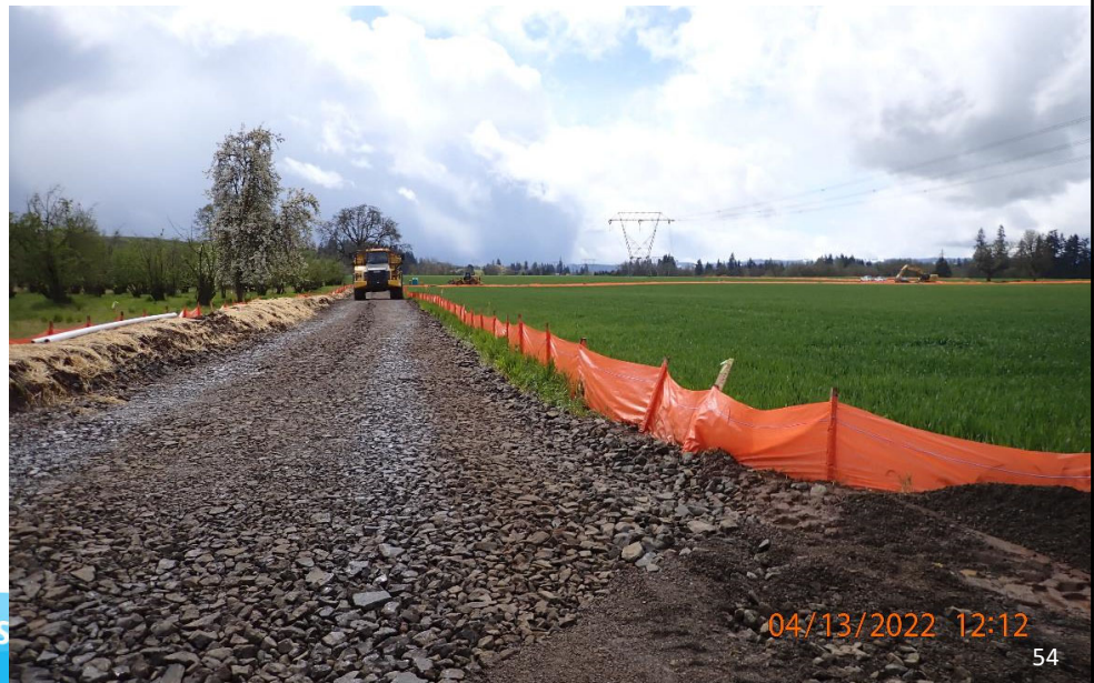
Temporary haul road construction
