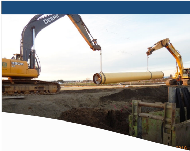
Construction of the additional water supply
