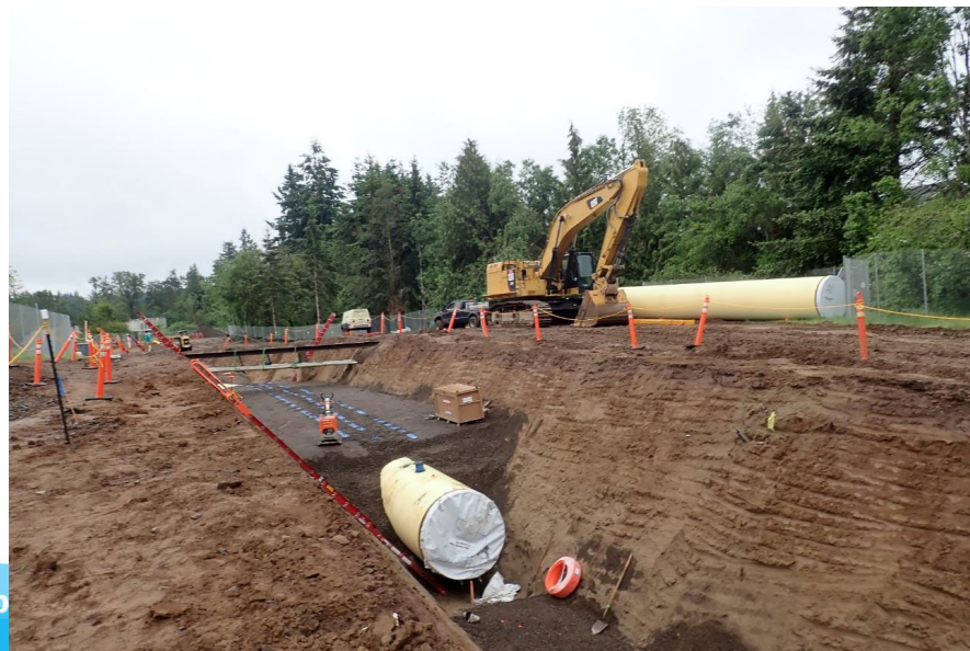
66-inch Raw Water pipeline progress through park
