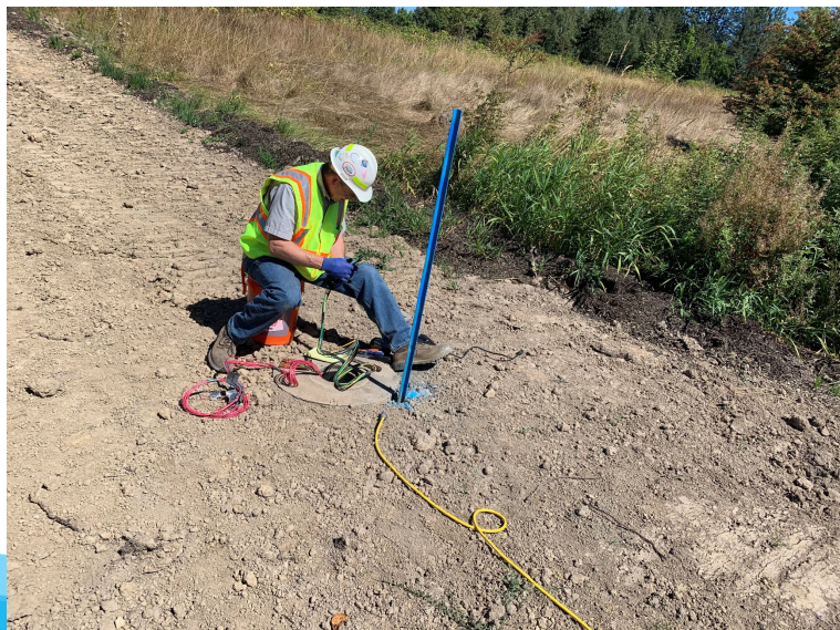
Cathodic Protection Test Station Install
