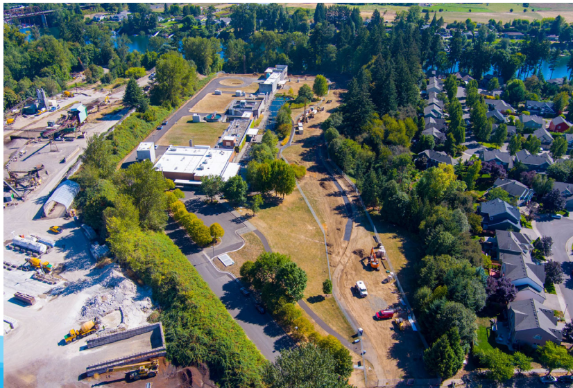
Lower Site pipeline corridor and temporary access road construction
