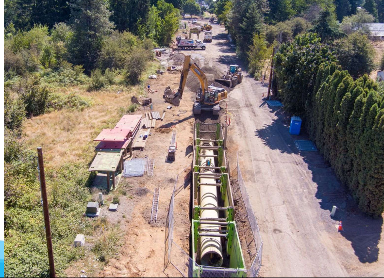
Waterline installation on Garden Acres Rd.
