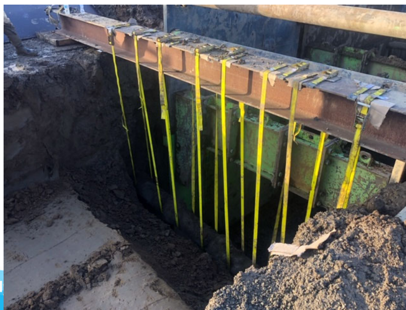
Protection of Sewer Line Crossing the Trench
