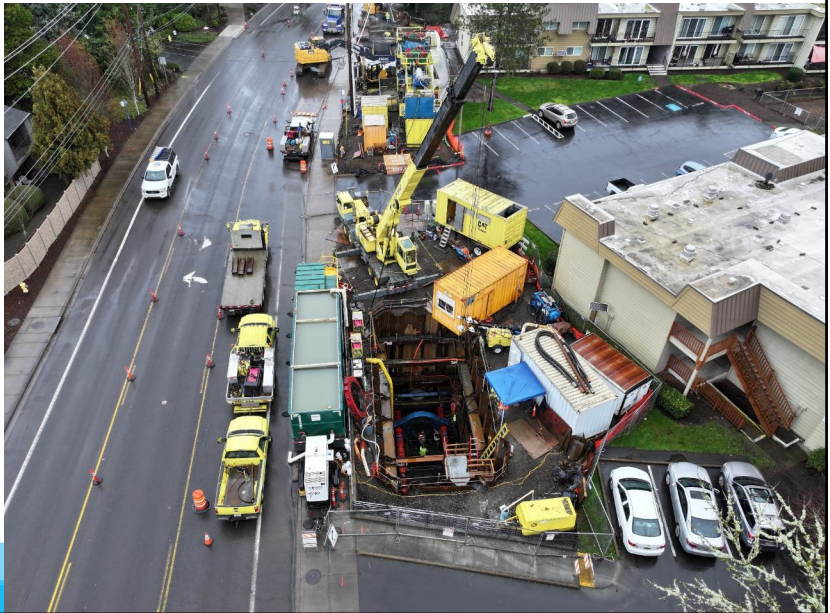
Upper Fanno Creek trenchless crossing site
