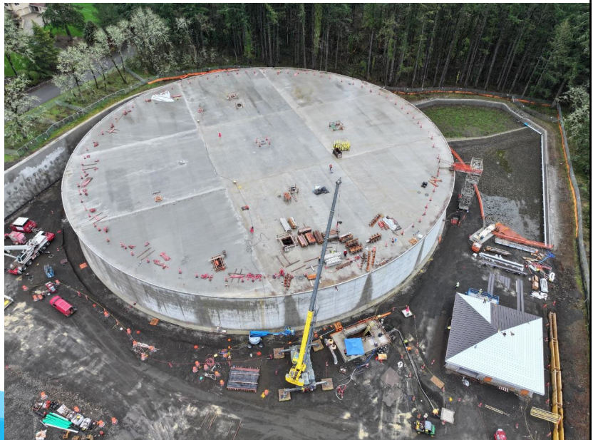
Reservoir concrete roof installation complete. Water Quality Bldg. under construction
