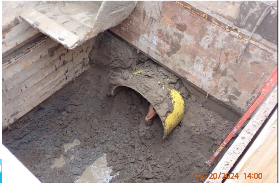
Tunneling head breaking out at receiving shaft at corner of SW Boeckman Rd. and SW 95 th Ave.
