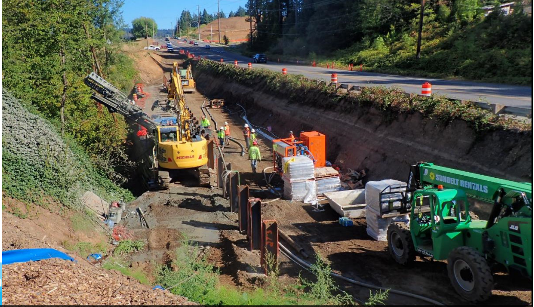
Installation of retaining wall at Tributary #4
