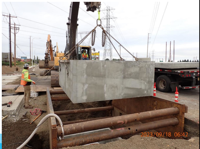
Setting precast concrete access vault.
