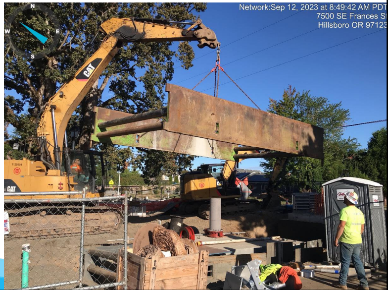
Frances Street turnout vault and piping construction
