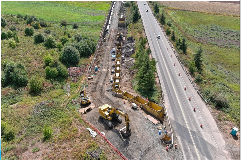
Open cut waterline construction on east side of Roy Rogers Rd.
