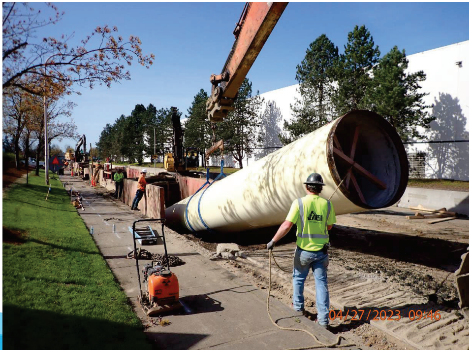
66-inch pipe installation on 95 th Avenue
