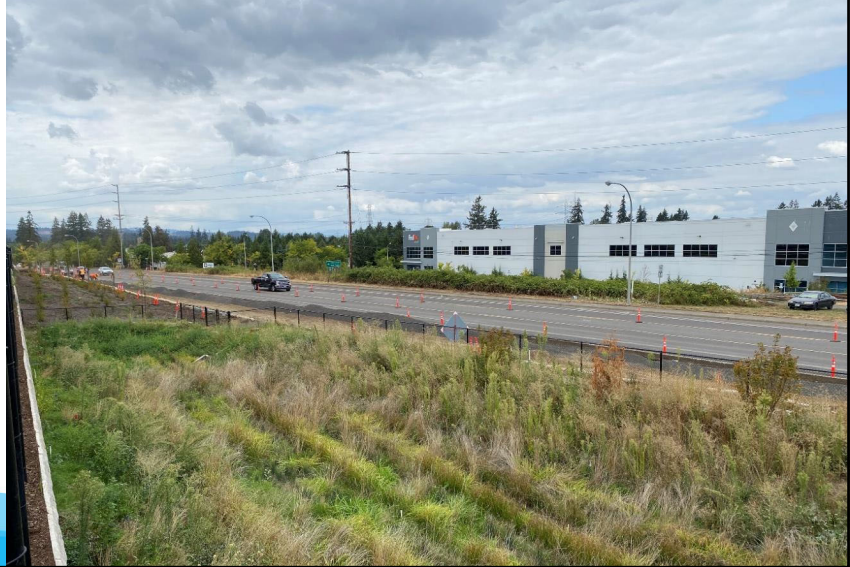
Road work along Tualatin-Sherwood Road
