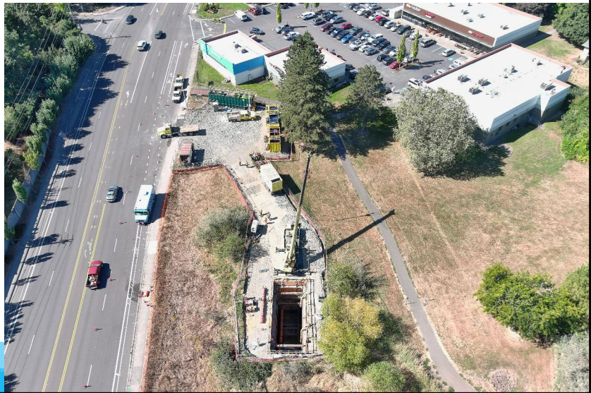
Tunnel #1 launch shaft near Greenway Park and Fanno Creek Trail
