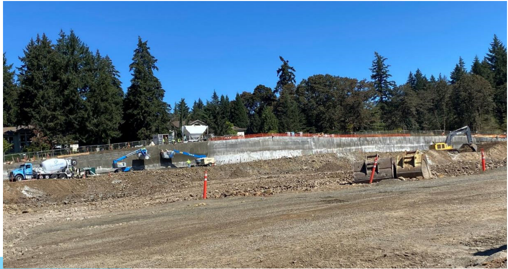
Excavation and shotcrete application at RES_1.0 site
