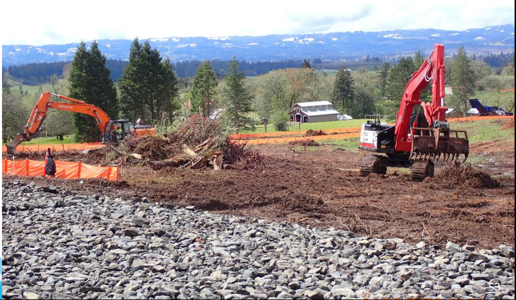
Grubbing on Staging Area #1
