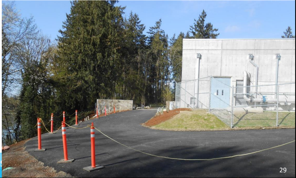
Raw Water Pump Station, permeable asphalt access road
