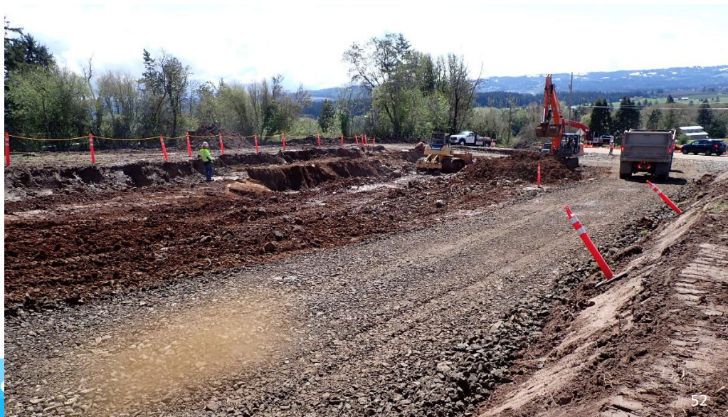
Initial earthwork at RES site
