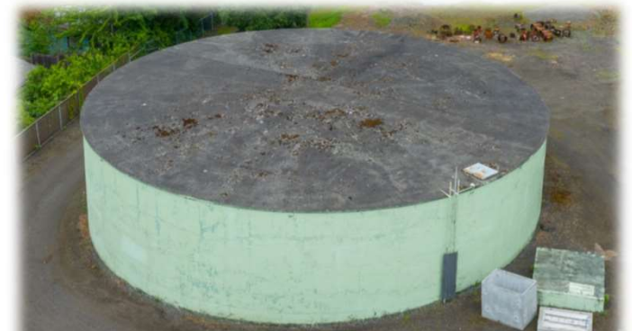
Taylor's Ferry Concrete Reservoir
