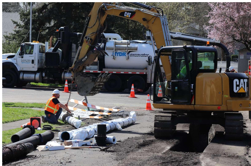
TVWD crews working on a main replacement project.
