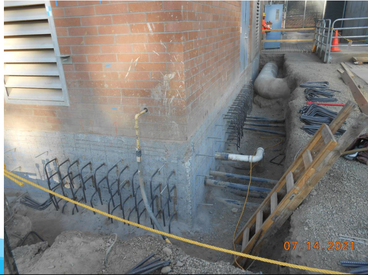
Seismic retrofit work at Raw Water Pump Station
