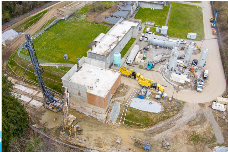
RWF_1.0 Lower Site aerial view. DSM and Jet Grout work occurring.
