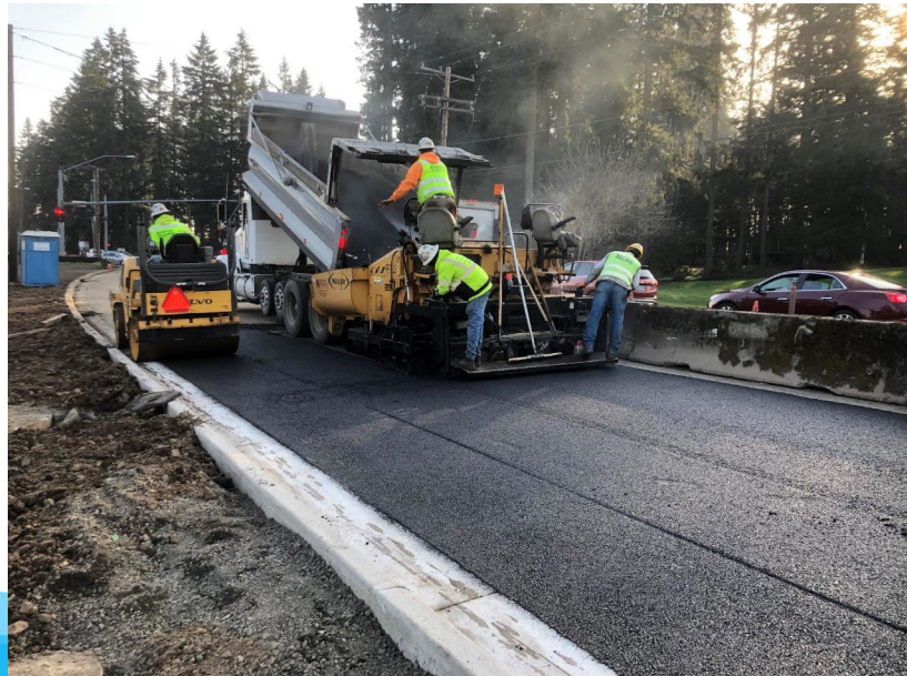
Paving Grahams Ferry Rd. after tie-in to PLM_3.0
