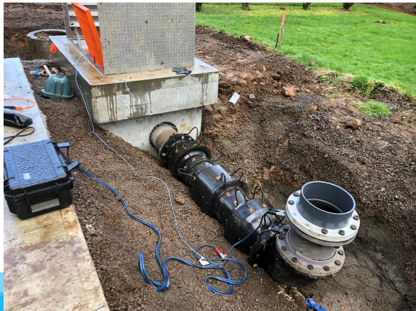
Type II CARV Vent Piping Installation
