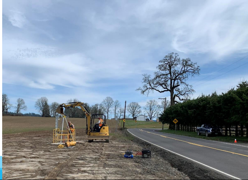
Installation of Vault Ladders
