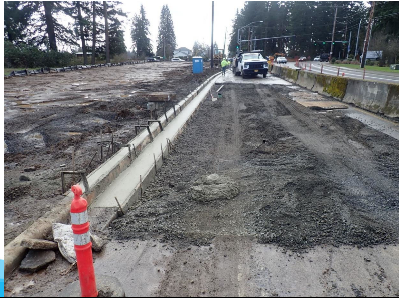
Curb and gutter replacement along Grahams Ferry Rd. at Tie-in point
