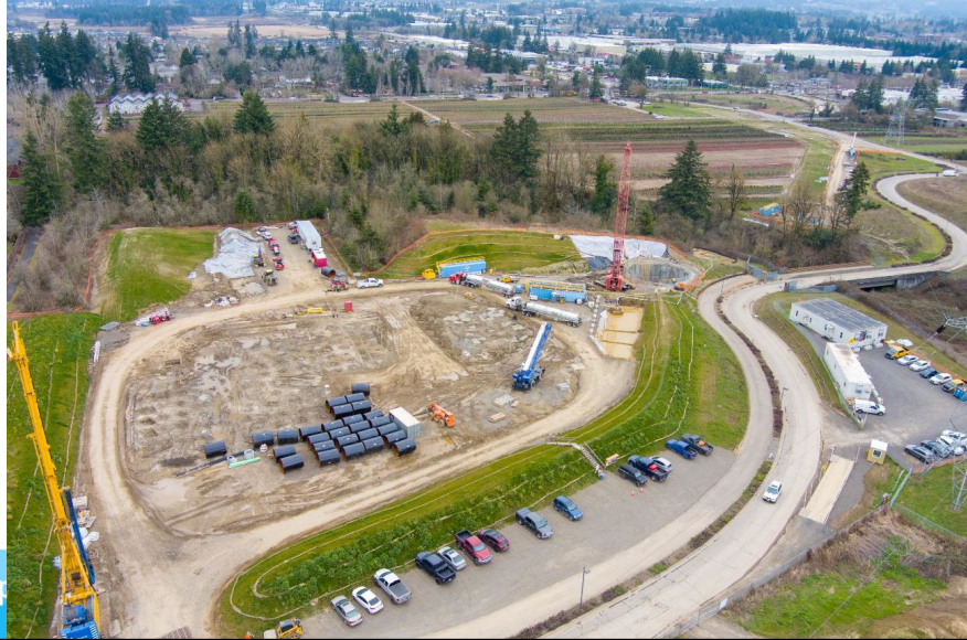
RWF_1.0 Upper Site aerial view
