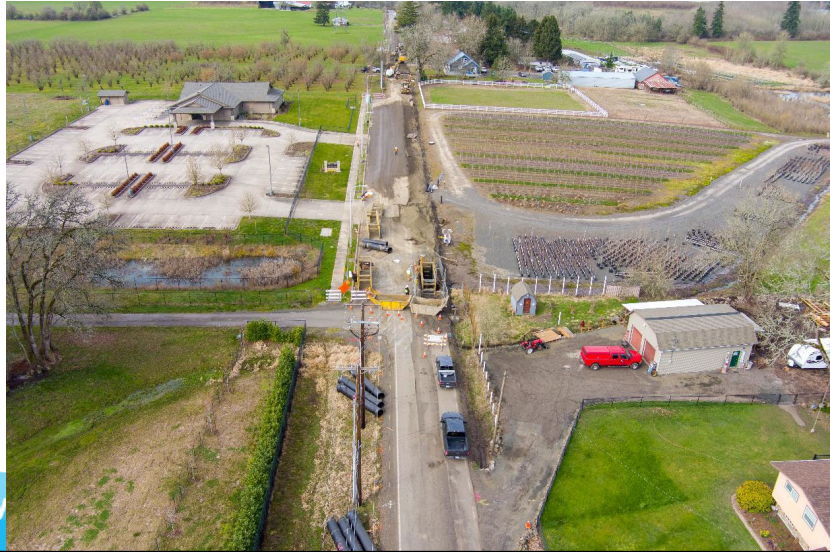
30-inch ductile iron pipe on Rosedale Rd. (looking west)
