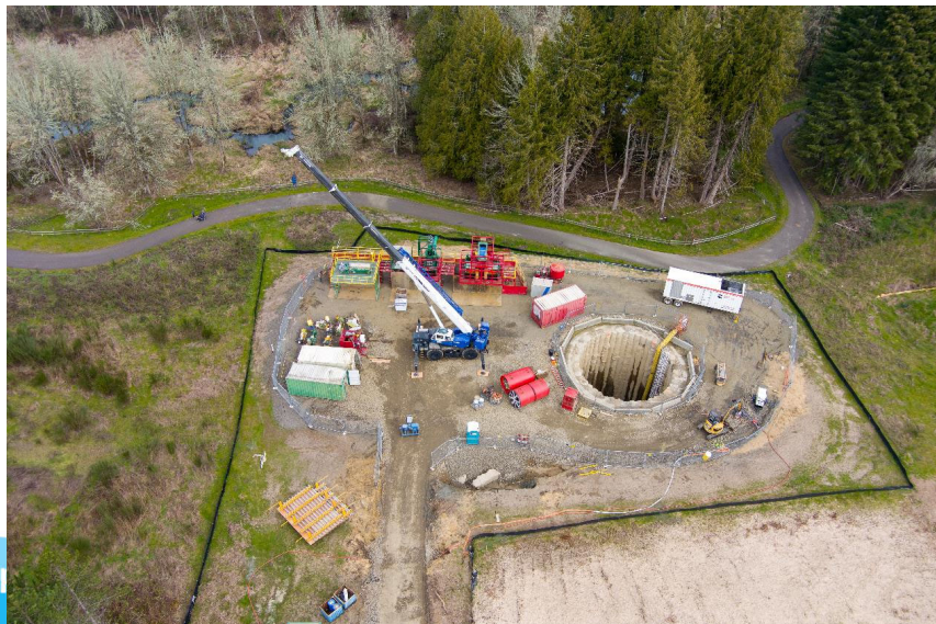
Microtunnel launch shaft. Tunneling equipment mobilized.
