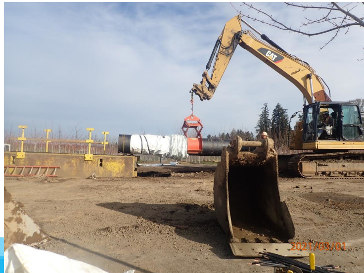
30-inch ductile iron pipe on Rosedale Rd.
