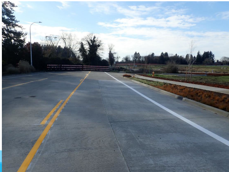
Final roadway striping repair on Kinsman
