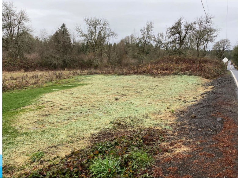
Erosion Control at Project End
