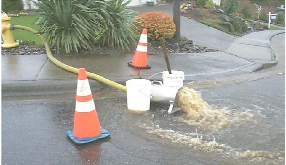
Every so often, TVWD staff open fire hydrants around the District and allow the water to flow through the pipes. Our hydrant flushing program is very important to our water system. It is an integral part of our ongoing effort to deliver the safest and highest quality water possible. It serves the following purposes:
