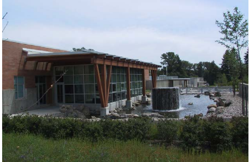
Pictured: Willamette River Water Treatment Plant
