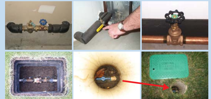
Your water shutoff can be one of many different types of valves. You can also shut it off at your backflow device.
